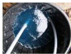
Fig 27 Slinkies Purged of Air
