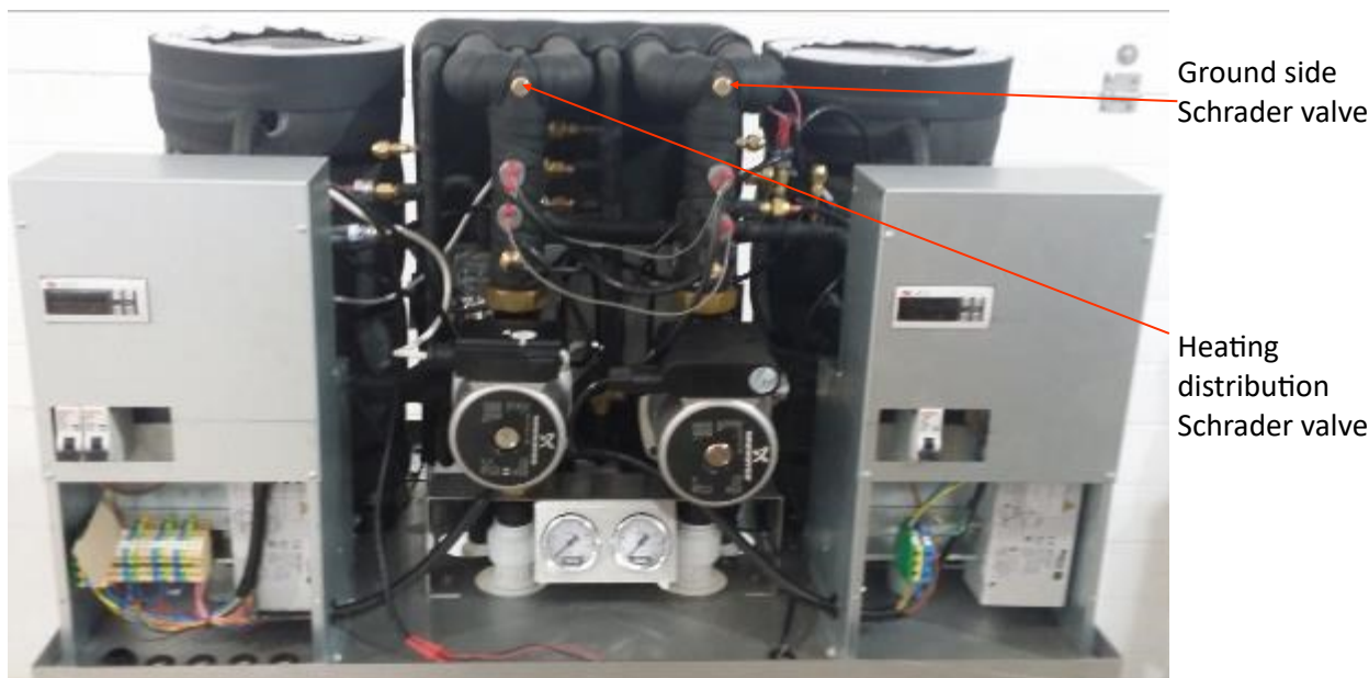
Fig 30 Location of Heat Pump Schrader Valves
