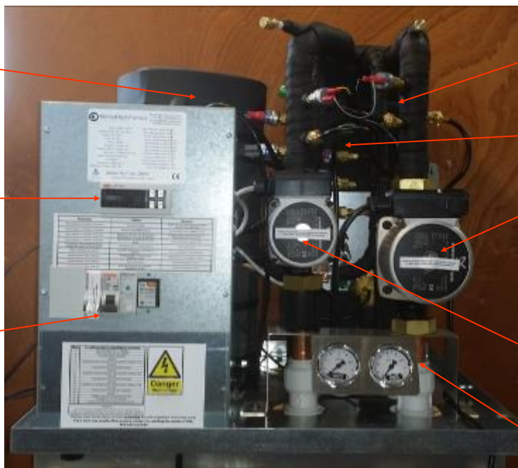
Fig 1. The internals of a heat pump
