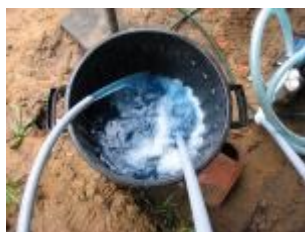
Fig 30 Purging the Slinky of Air
