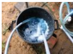
Fig 25 Purging the Slinkies of Air
