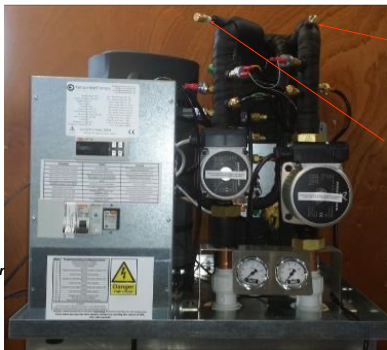
Fig 32 Location of Heat Pump Schrader Valves
